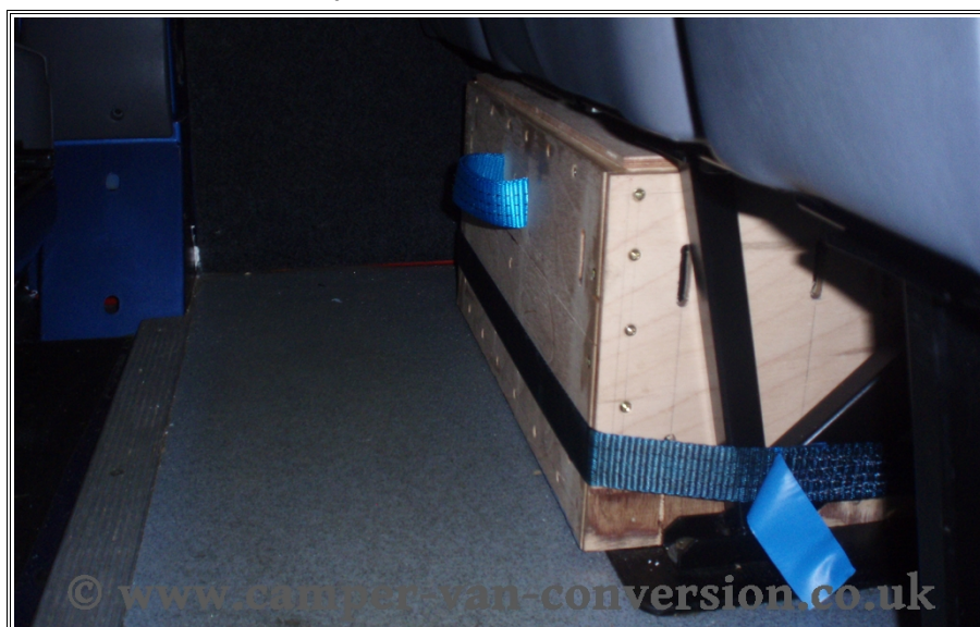
Battery box secured under the seat.
